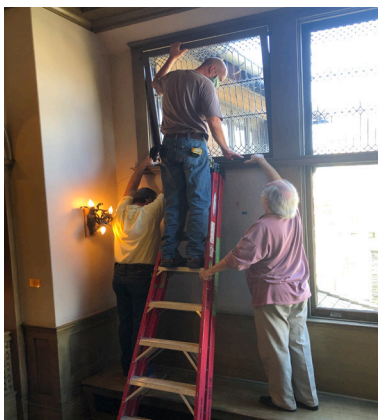
WSU carpenters and Freer House board member, Doug Peters, install a restored leaded glass window
