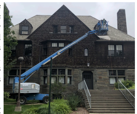
Restoration of 3rd floor dormer windows
