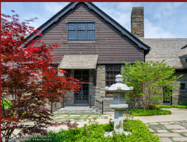
Exterior view of the former location of the Peacock Room at the Freer House. Photo by Alex Vertikoff, 2022.
