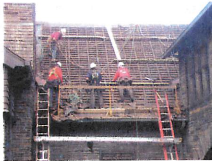
(roof under construction)
