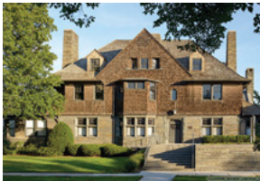
THE FREER HOUSE The historic 1892 Freer House has proudly served as home to Merrill-Palmer since 1920.
